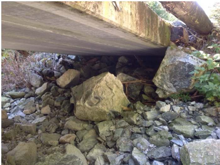
Right Bank Abutment when facing downstream
