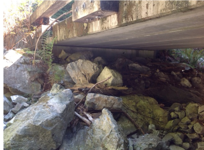
Left Bank Abutment when facing downstream
